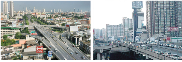
Figure 1: Borommaratchachonnani Elevated Road (image source: www.dailynews.co.th ).
